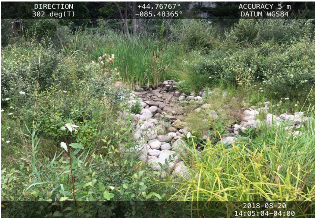
Photo 13: Basin # 1 swale outlet
