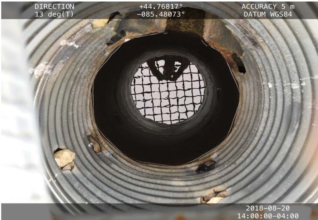
Photo 7: Basin # 2 outflow control structure (interior)
