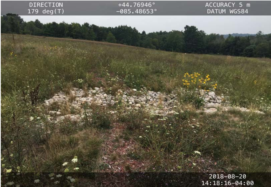
Photo 9: Basin # 2 emergency overflow
