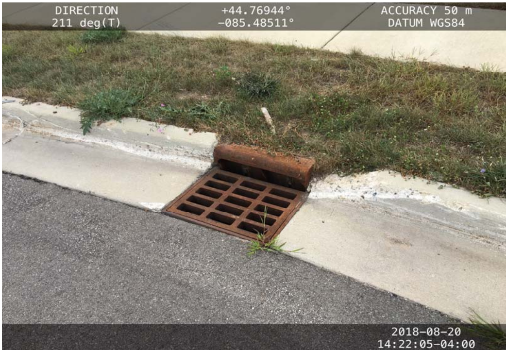
Photo 1: Catch basin inlet west corridor road
