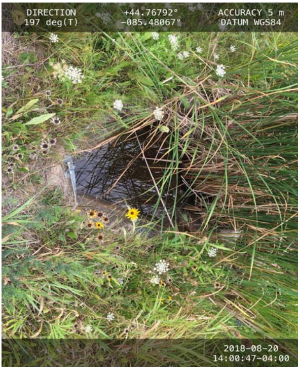
Photo 10: Basin # 1 swale inlet structure
