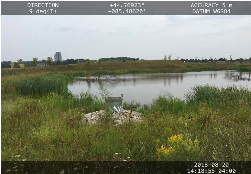
Photo 3: Basin # 2 detention pond viewing north
