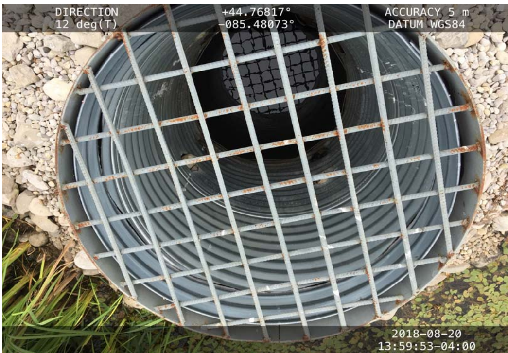
Photo 6: Basin # 2 outflow control structure (exterior)
