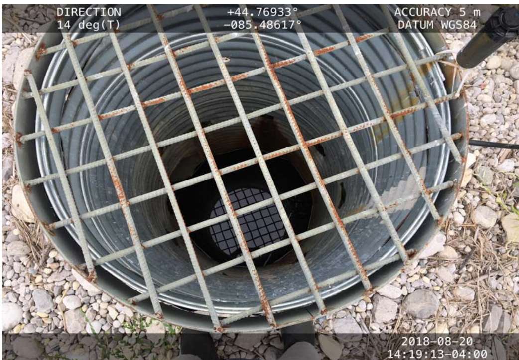
Photo 4: Basin # 1 outflow control structure (exterior)
